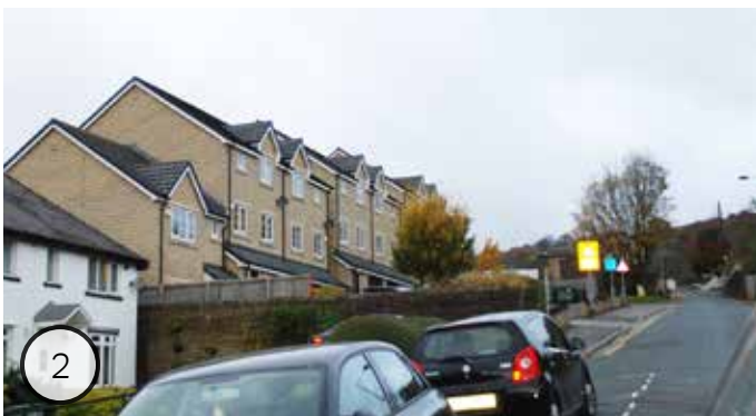
Parking spaces along narrow Micklethwaite Lane
