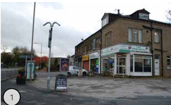
Poor quality public realm at the junction of Keighley Road and Micklethwaite Lane
