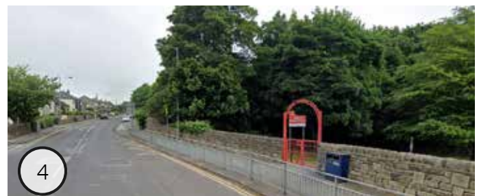
Unsafe and poorly arranged entrance for Eldwick primary school;
